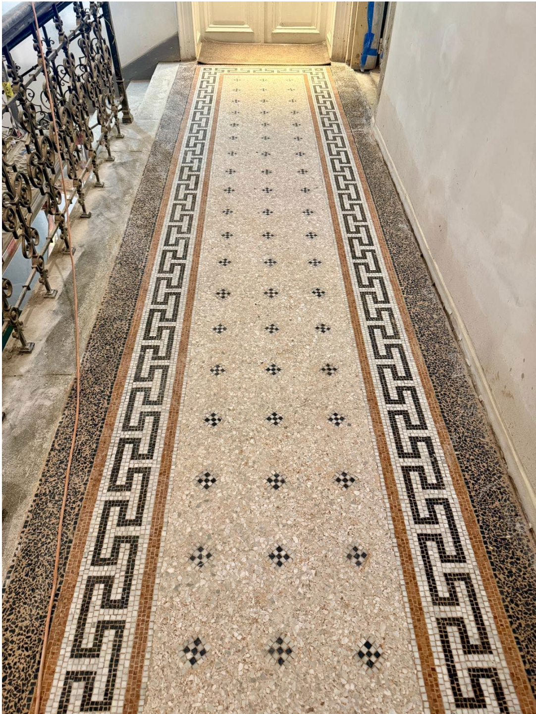
Detail Terrazzo-Boden Treppenhaus
