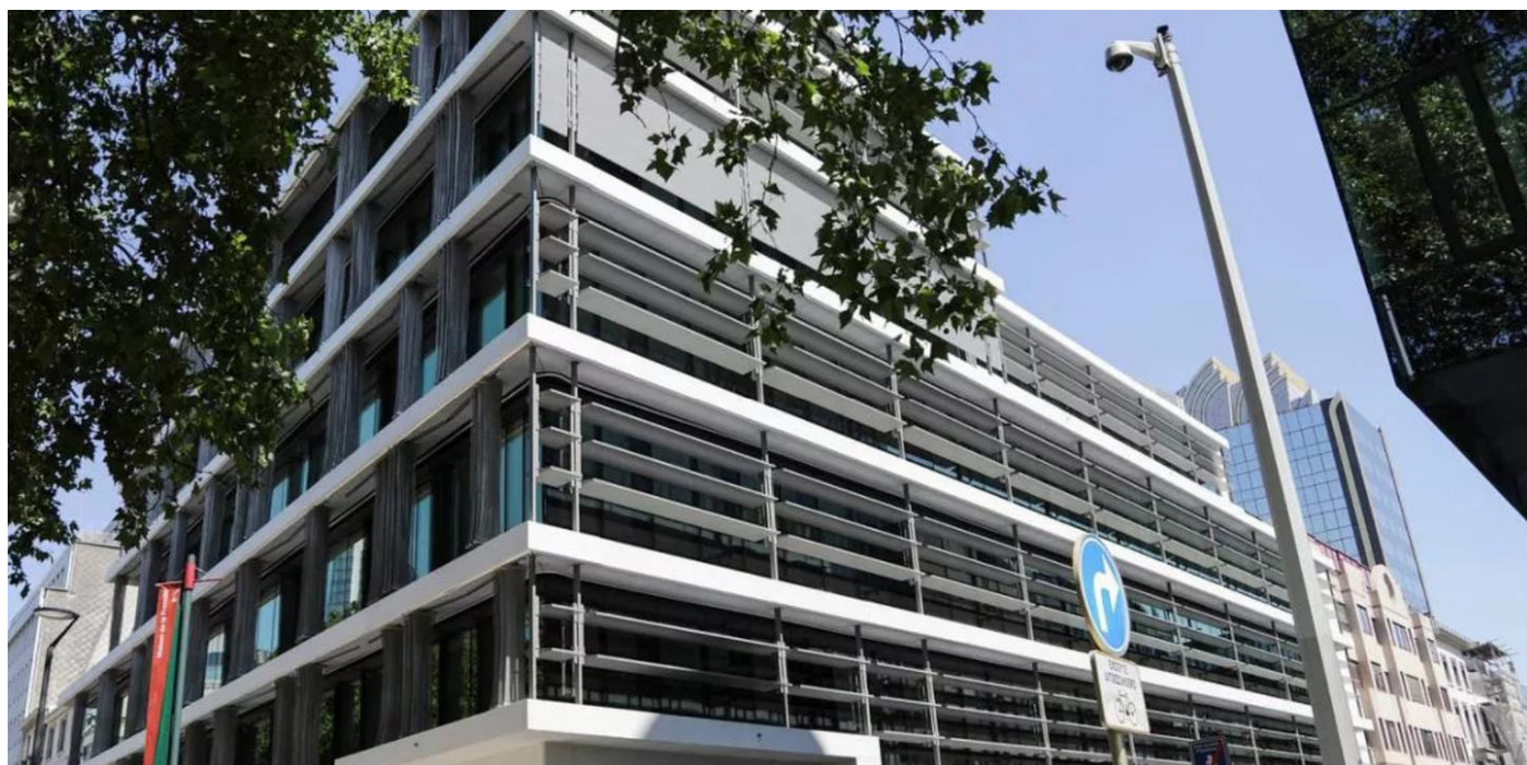
In March 2021, ESA moved into its new headquarters in EFTA House. The office building is shared with the EFTA Secretariat and the Financial Mechanism Office.
